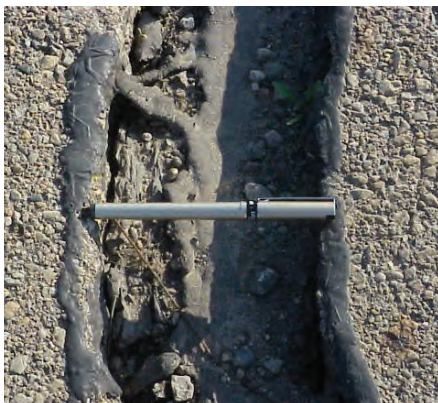
Failed Crack Seal = BIG Safety Hazard
